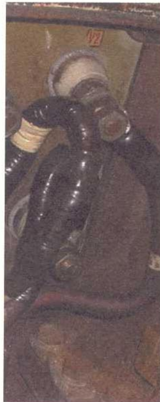
Detail of fire pump electric terminal box and corresponding thermophotograph.
